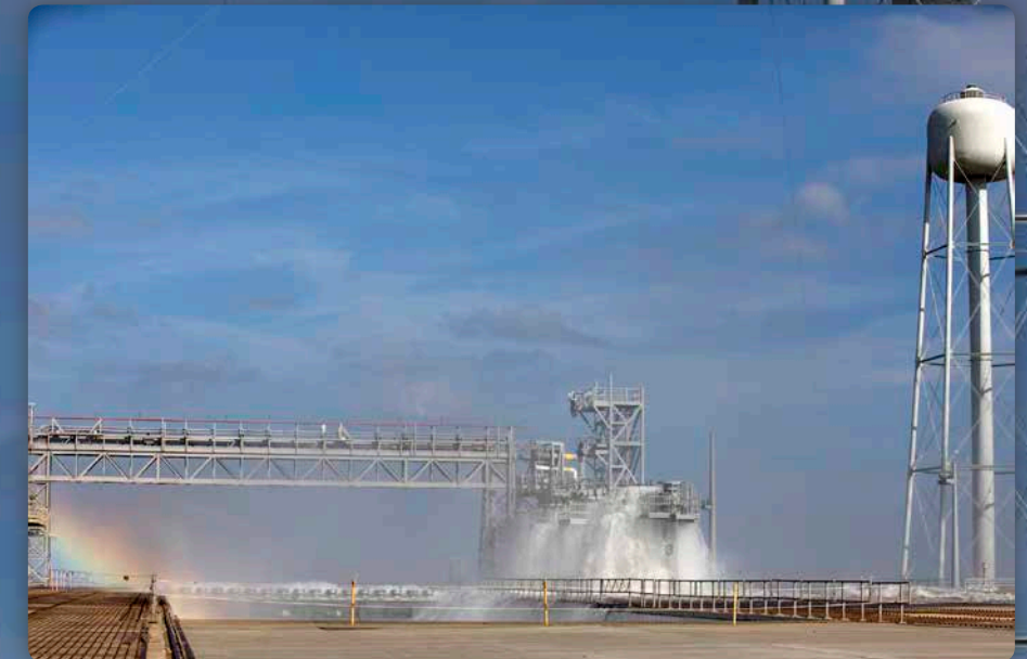
Water flowed at high speed from a holding tank through piping and valves, the flame trench and mobile launcher interface risers during a wet flow test at Launch Pad 39B at NASA's Kennedy Space Center. Photo credit: NASA/Kim Shiflett
